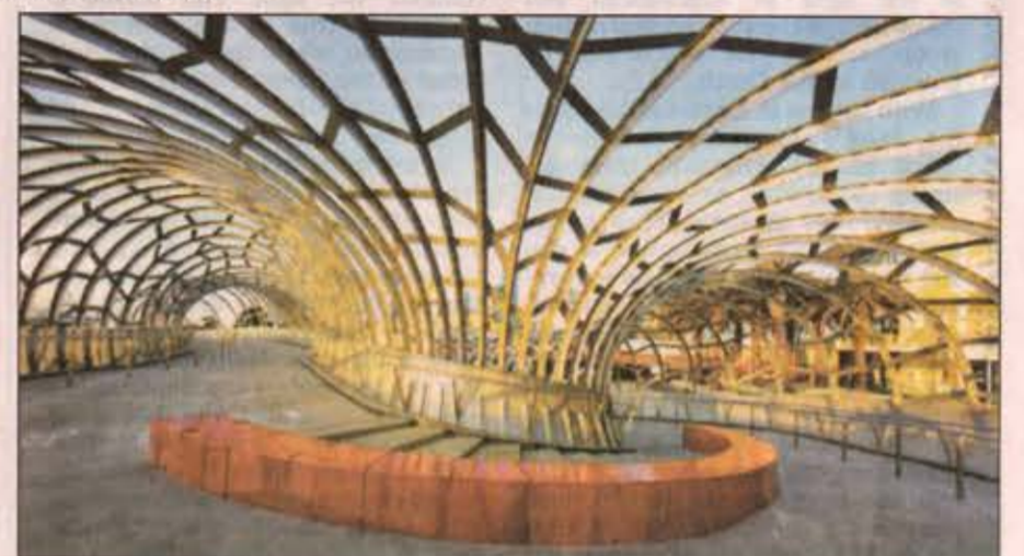
Total structure: Architect and artist worked together on Melbourne's Webb Bridge
